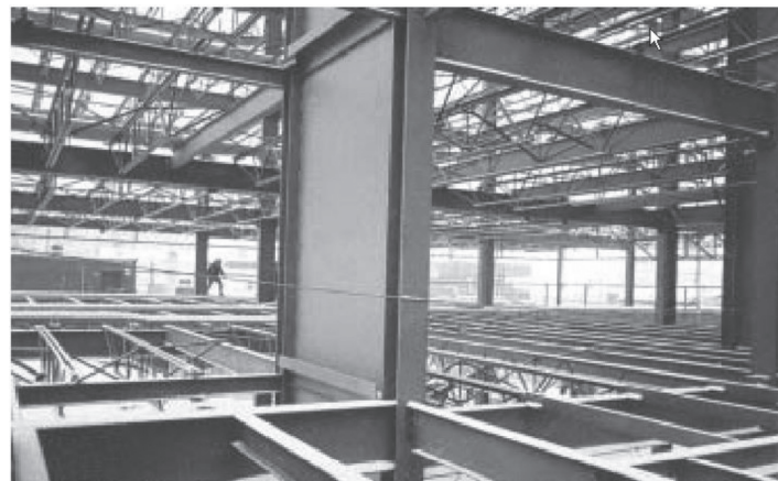
FIG. 17.41 Planar SPSW system of the Canam HQ building, Canada
