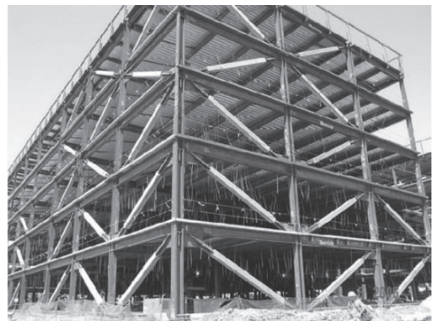
FIG. 17.47 BRBF at Kaiser Permanente Hospital, Vallejo, CA. Reprinted with permission, STRUCTURE magazine, February 2008.
