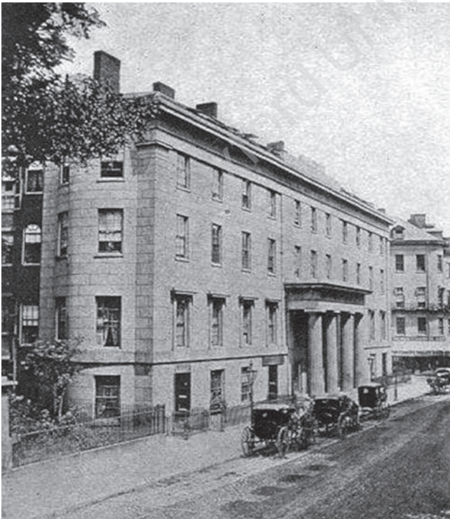
Figure 1.13 Tremont House, Boston
